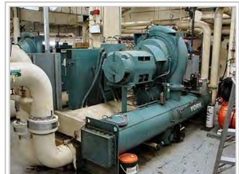
Figure 5: Commercial water-cooled liquid chiller installation for building air conditioning
